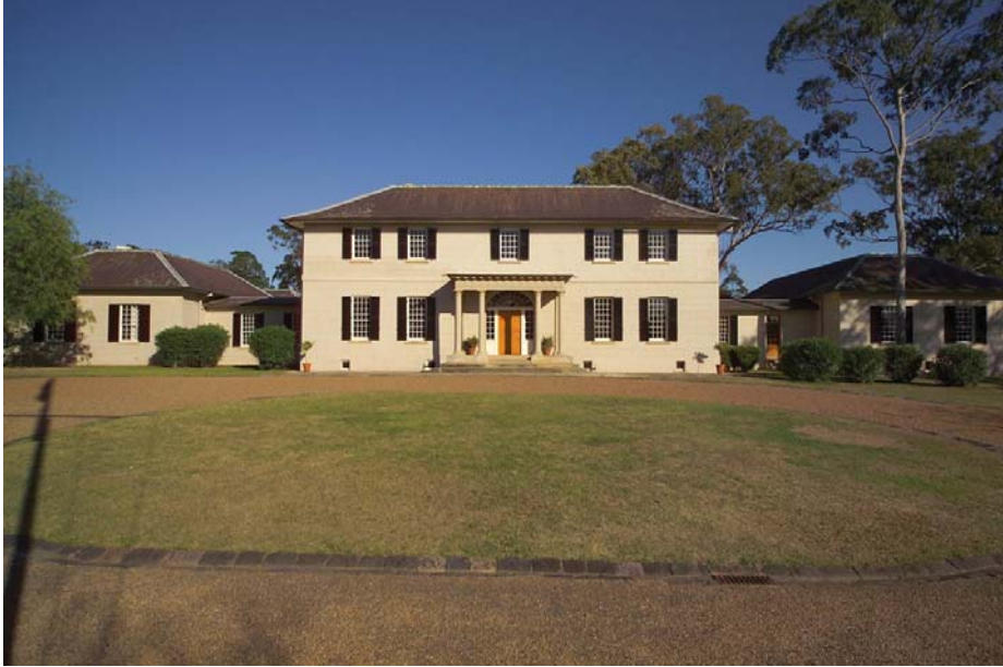
Figure 12: Principle façade of Old Government House indicating current state of conservation following works in the 1993-2001 period. (Source: National Trust, 2006)
